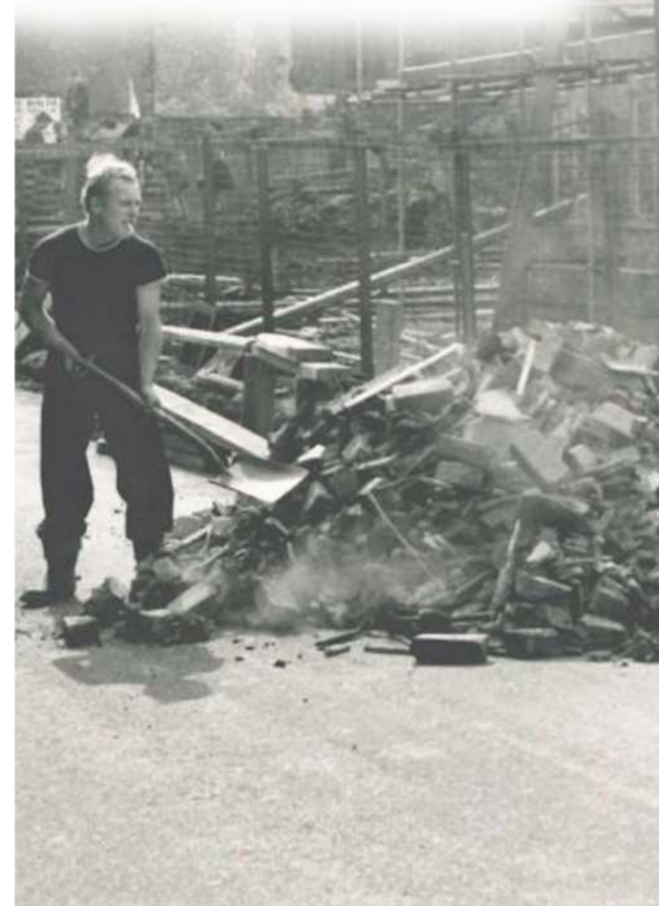
Fig. 17 Building work and the older terraced housing in the Groves
